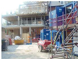
Progress on the new Dacre Block is continuing apace. The steel frame is now complete and the concrete floor has been poured. The brickwork should be completed around the end of September and then work can commence on the roof. Buxtons is due to hand over the building to the School by December 2016.
