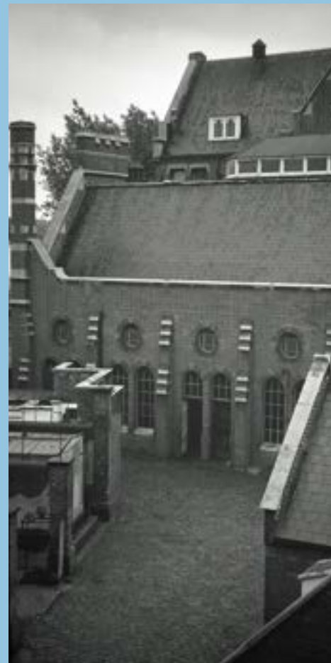
2. Room 11 eventually demolished
