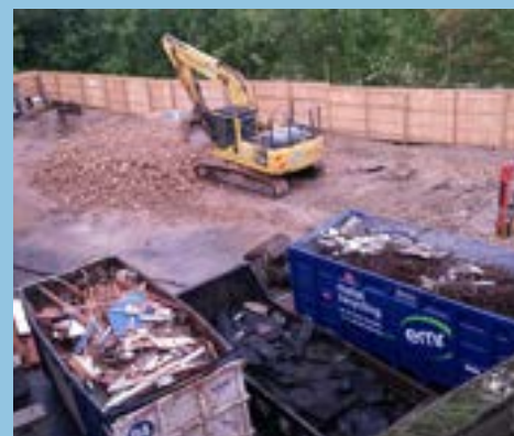
6. Setting the foundations for the New Dacre
